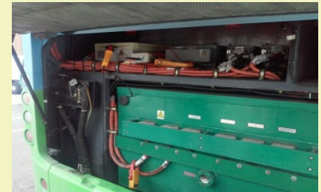
Measurement of the current consumption of the system for heating the passenger compartment
